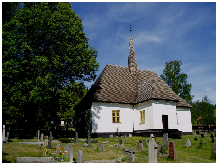
Fig. 11: Djurö Wooden Church, Sweden
